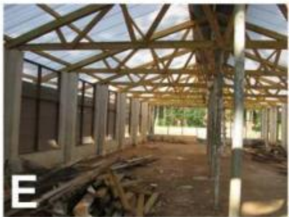
Figure 6. Facilities at Chitedze Research Station (A); the current biotechnology lab (B); the new facilities (C,D) and green house in progress (E).
