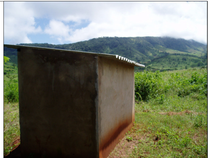
Fig A10.10: Toilet block at Family Sector Farm near Vanduzi
