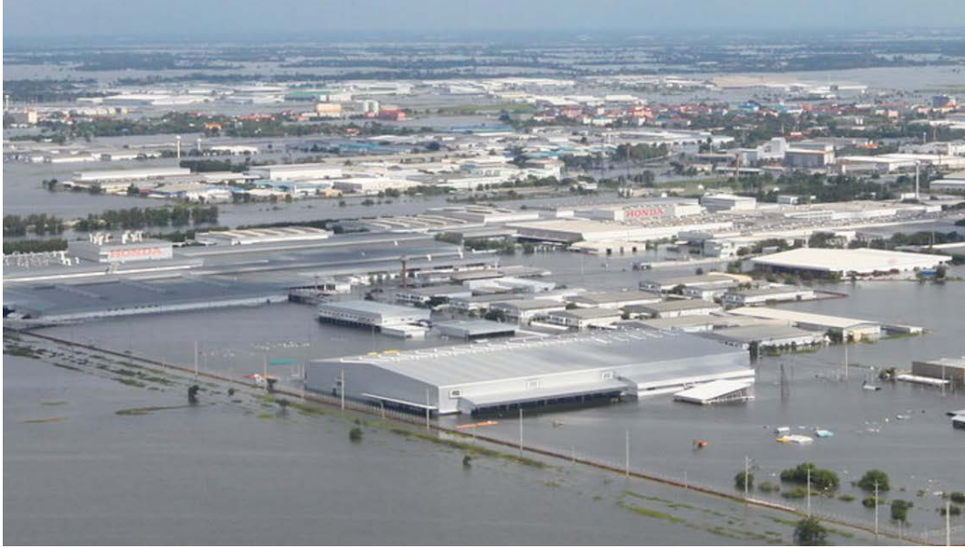
Fig. 3 Flood Inundation at the Rojana Industrial Park, Ayutthaya Province
