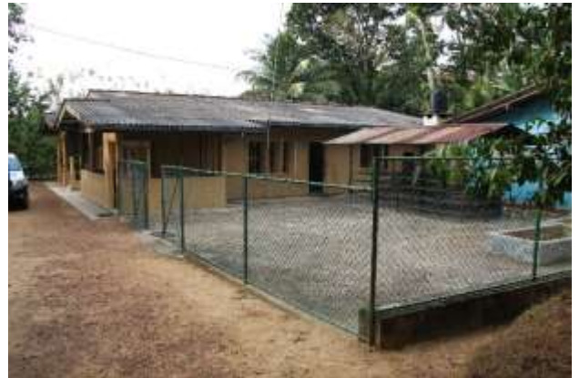
Figure 7. View of outdoor washing and drying area of factory
