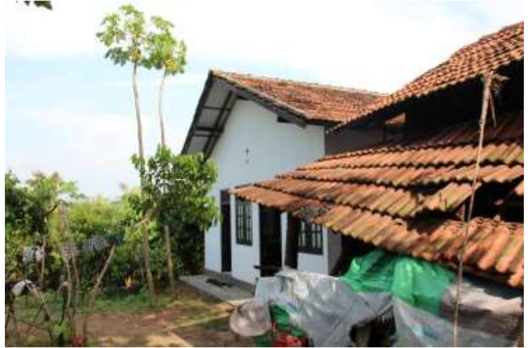
Figure 14. Back side view showing separate entrances to scrapping section and room used for resting and office work
