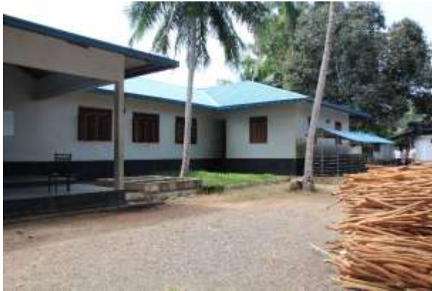
Figure 1. Front elevation view (part of building from left side)
