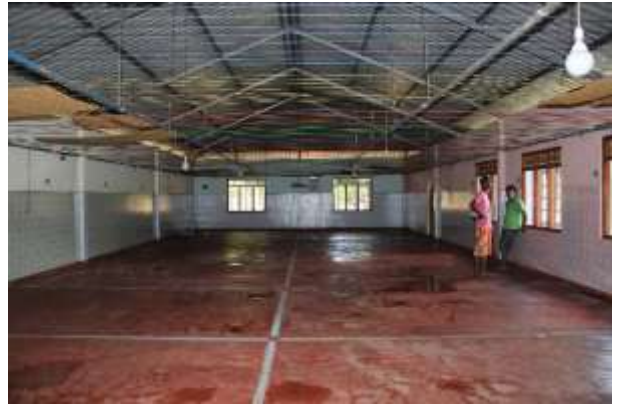
Figure 2. Interior view of building (from left to right)
