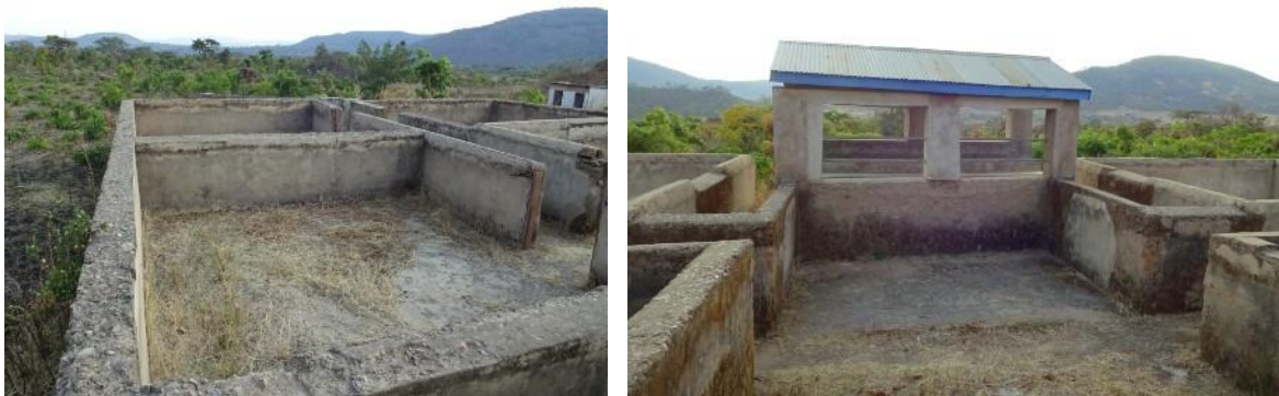
Figure 7. The holding pens and bidding area for the new official Kasesya border market (under development during visit in autumn 2016)
